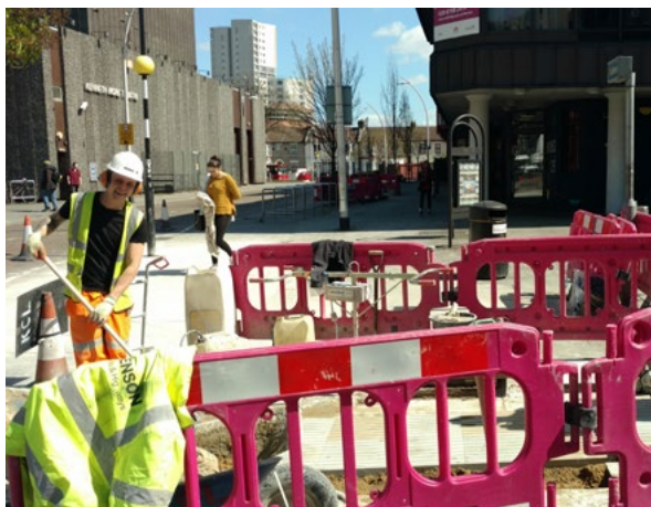
Street maintenance and repaving
