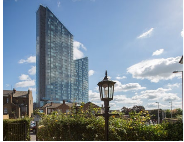
Pioneer Point, Winston Way Junction, Ilford
